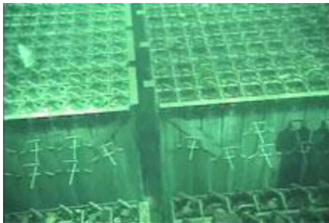
Figure 2. Dense-packed spent fuel in the spent fuel Storage pool of Fukushima Daiichi Unit #4. 24
